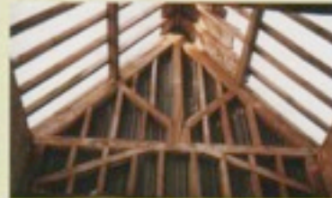
Internal Woodwork Prior to Removal
