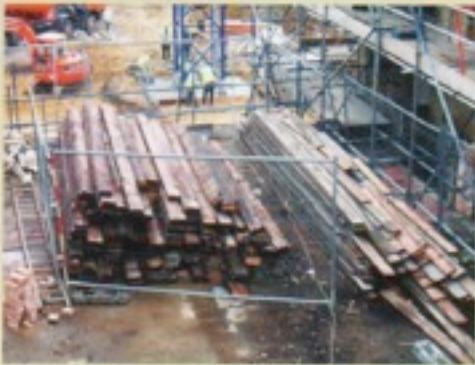
7 tonnes of timber reclaimed from the houses in Putney including joists, floorboards and doors
