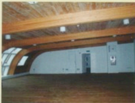
Reclaimed timber floorboards used for floor and ceiling finish at Jubilee Wharf
