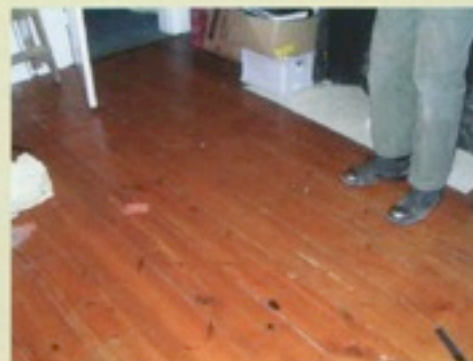
Timber floorboards found throughout the property
