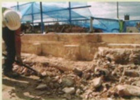
Clearing rubble to expose face stone
