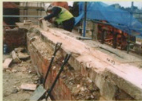
Numbering of stones before removal
