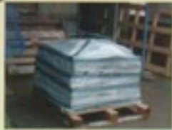
Face stone measured, catalogued and inventoried onto pallets
