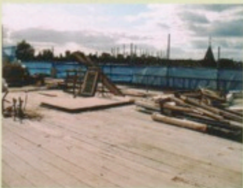
Floorboards to be lifted, August 2006
