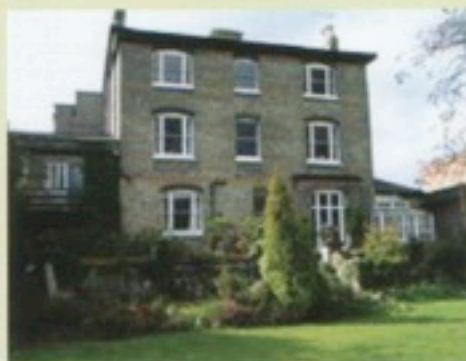
Putney house prior to demolition
