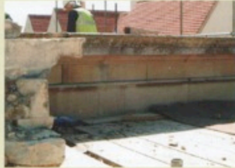
Parapet wall, right wing, main facade
