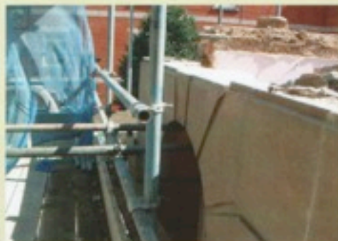
Left front door – scaffold poles used to support stone during dismantle
