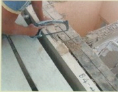
Cutting out the steel ties from the stone
